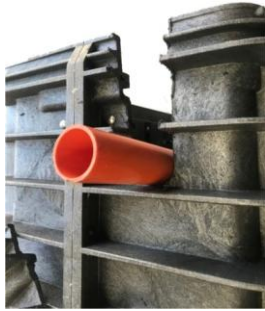
Example of conduit positioned in a top cut mouse hole
