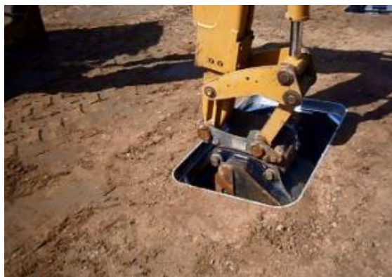
Fig 30: Manhole Cell Compaction
