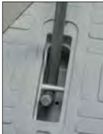
Recessed Lifting Pin with Cover
